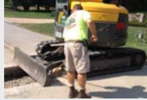
Denny Miller repairing the culvert on Huffman Road
