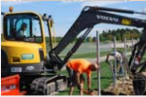
Service Dept. preparing dugouts for cement at Blakslee
