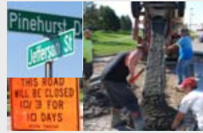
Road Repairs at Jefferson and Pinehurst Drive
